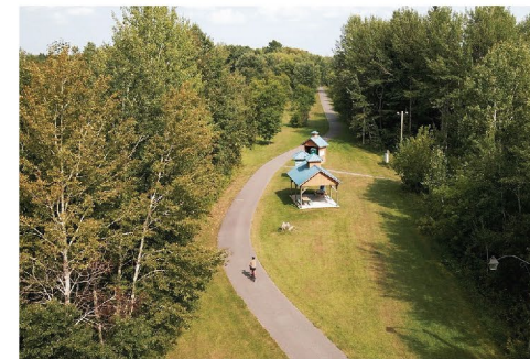
Construction of a toilet shelter
